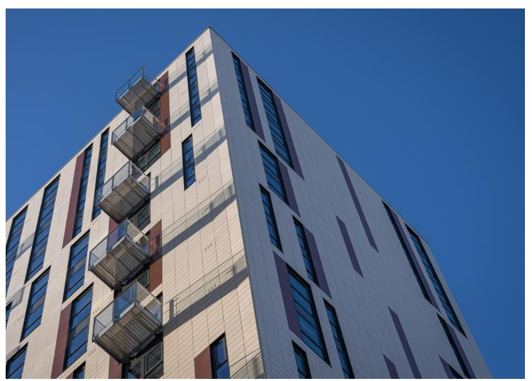
Two types of Kawneer's zone-drained curtain walling – AA®100 with 50mm sightlines and AA®110 with 65mm – as well as AA®541 top-hung casement windows and thermally superior AA®720 balcony doors were specified by AHR architects for Plot A7 at The Slate Yard.
